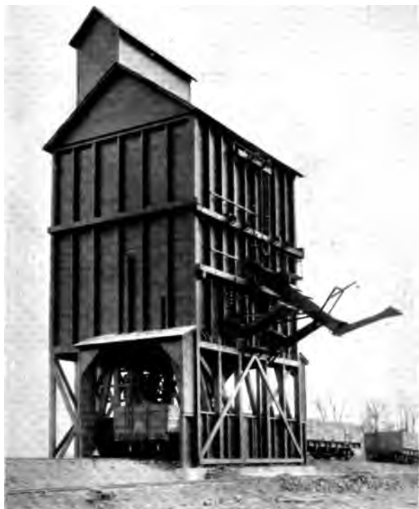
Coaling Station of Timber Construction Serving two tracks on one side
